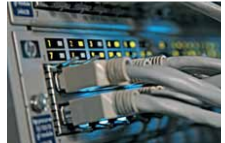
Technical infrastructure completely reworked
